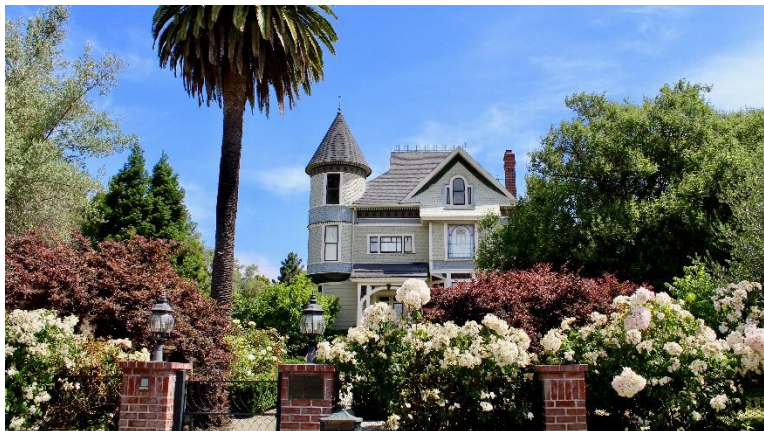
Historic Victorian House
