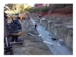
As a result of continued monitoring of the western slope below Silver Oaks Townhomes, the GHAD has made a determination that it is advisable to install slope stability measures to prevent future movement of the slope. Engineering and construction documents have been completed to define a slope stabilization scheme similar to those utilized in the area. Work will proceed pending landowner authorization to allow access to the site.
