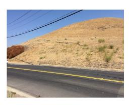
A late season landslide emerged along Blackhawk Road (near Lacrosse Field). Slide margins threaten the roadway below on Blackhawk Road. Winterization measures were taken, and design and construction documents have been generated. Work is expected to occur in FY18/19.
