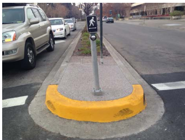
Photo 18 Pedestrians can wait in the middle of the roadway if they started crossing late in the phase and did not make it across before the end of the phase. While the pushbutton is in reach of wheelchair users, the relatively narrow median and lack of protection from turning vehicles makes it an intimidating place to wait.
