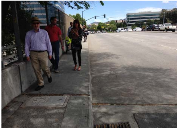
Photo 6 View east along the existing 5' wide sidewalk on the I-680 overcrossing. Pedestrians are observed walking in the traffic lane to overtake one another.
