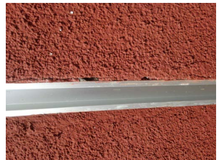
Small gaps in stucco that had to be filled on the exterior of Bldg 500 at 255 Glacier in Martinez to prevent cockroaches from getting in.
