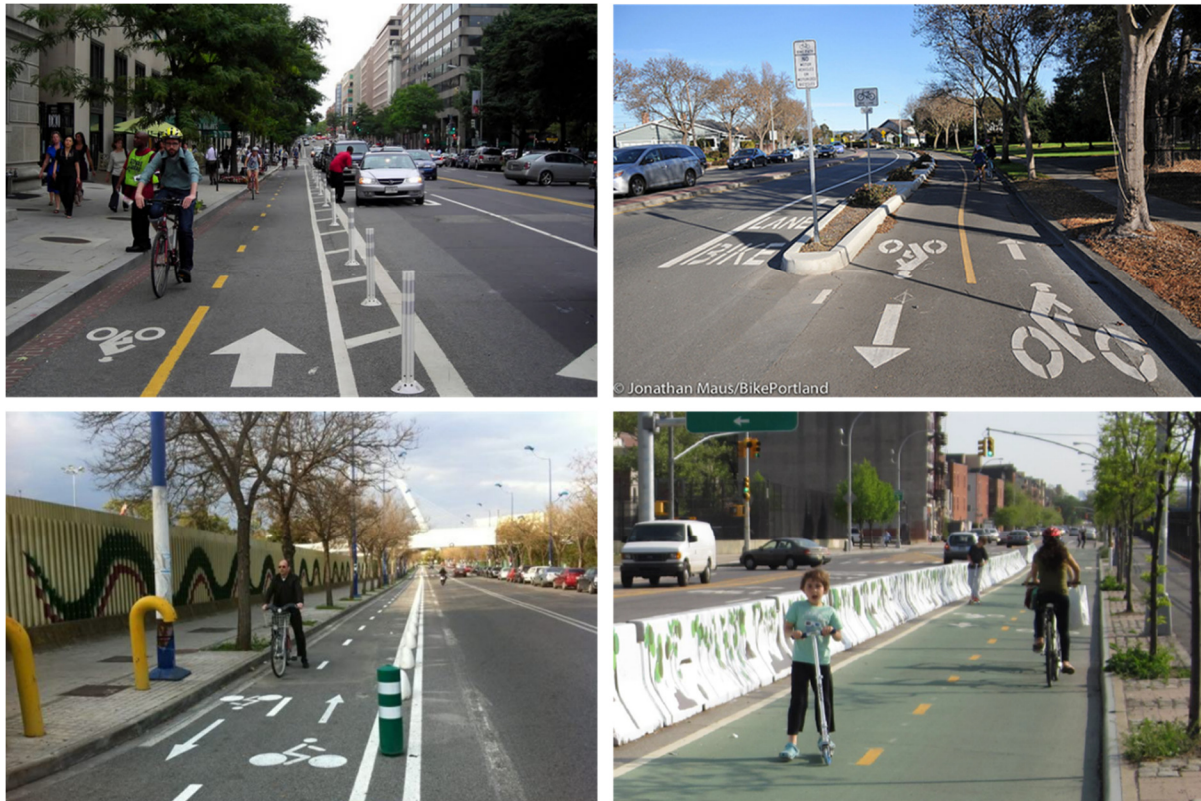
Clockwise from top left: flexible pylons and striping; curb and gutter island; Jersey barrier (“K-Rail”); and inflexible bollards
