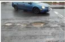
Pavement – The last 5 years have been kind to us regarding winter weather. However, this year's storms are exposing the poor condition of our pavements. Water is the pavements worst enemy if it reaches underneath through cracks and worn surfaces. These small cracks can lead to big potholes very quickly when exposed to wet weather.
