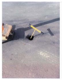
Sinkhole in the roadway caused by road drainage pipe failing. We repaired a sinkhole on Hazel Avenue in East Richmond Heights. Several years ago we had a sink hole form on Marsh Creek Road that required immediate action to prevent the lane from collapsing.
