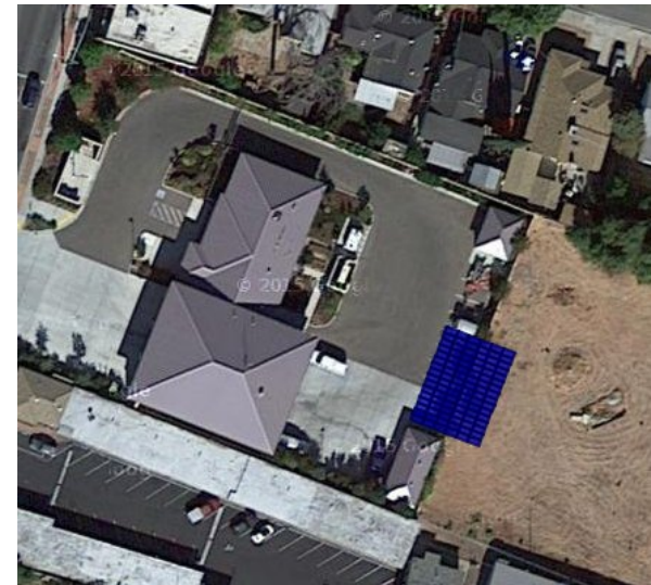
Fire Station 84 Pittsburg 33 kW
