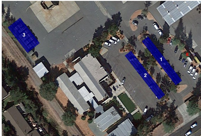
Fire Station 10 & Training Campus Concord 135 kW
