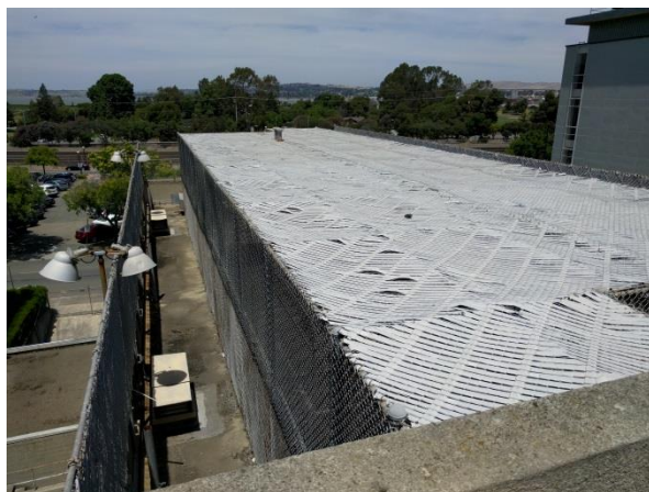
Photo 6. Roof of the annex with the chain-link enclosure.
