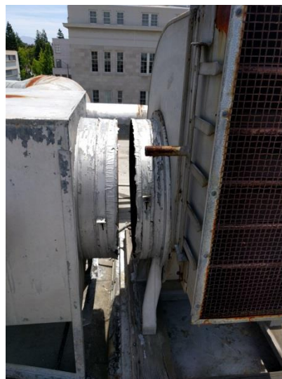
Photo 9. Opening in ventilation conduit.
