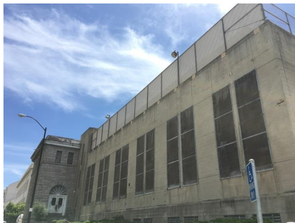
Photo 2. Concrete exterior of the annexed portion.
