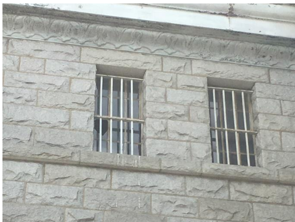
Photo 3. Night roost habitat under small overhangs and in corners of windows.
