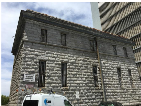
Photo 1. Granite exterior of the original jail.
