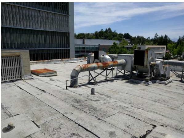
Photo 5. Roof of the original jail with external vents.
