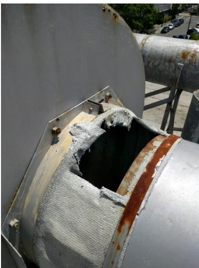
Photo 8. Opening in ventilation structure.
