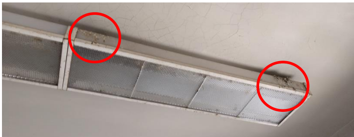
Photo 11. At least two active house finch nests on top of a light fixture on the top floor of the building.
