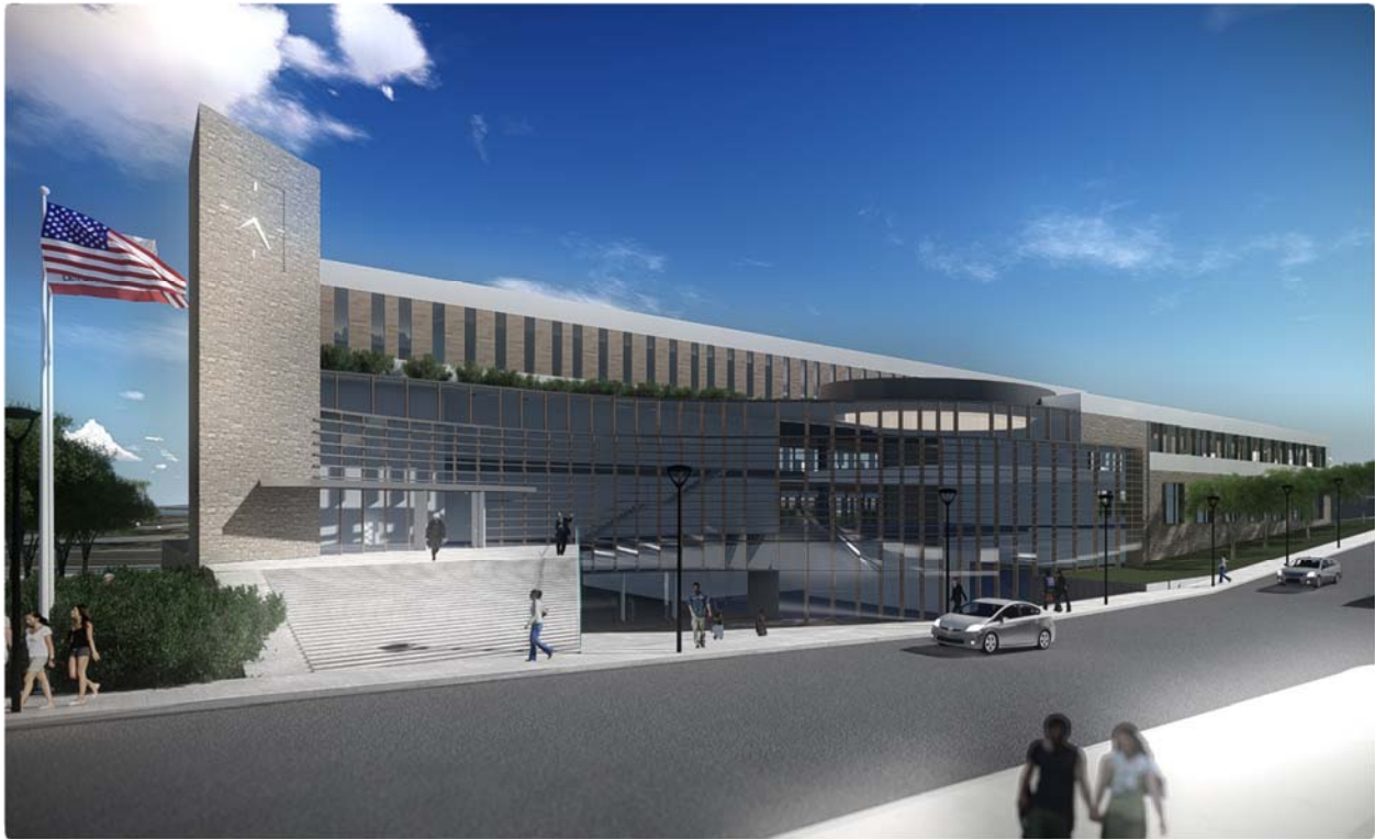
Figure 3 Main Facade New Admin Building
