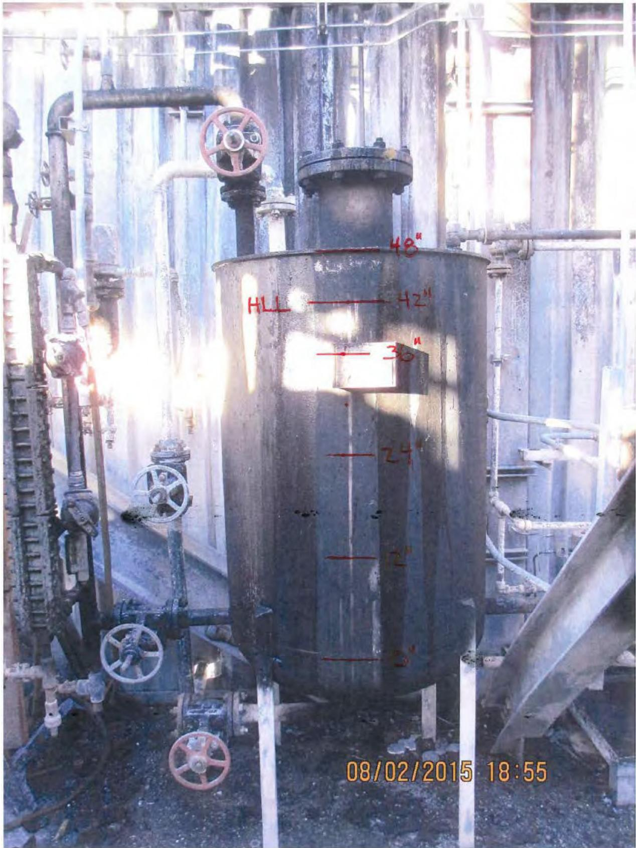
PICTURE OF DAY TANK WITH LEVELS MARKED
