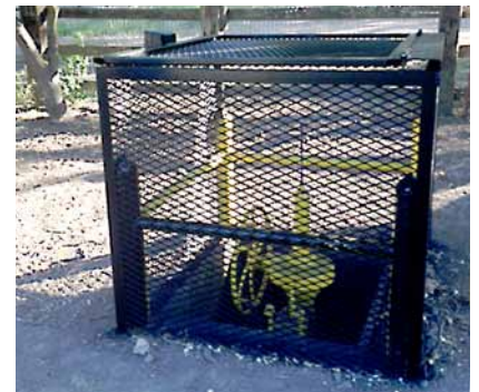
Manual valve inside protective cage in Alamo along Iron Horse Corridor
