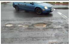
Pavement – The last 5 years have been kind to us regarding winter weather. However, this year's El Nino storms are exposing the poor condition of our pavements. Water is the pavements worst enemy if it reaches underneath through cracks and worn surfaces. These small cracks can lead to big potholes very quickly when exposed to wet weather.
