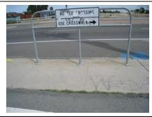
Road Signs – The County maintains hundreds of street signs. These must be checked routinely for reflectivity and replaced if necessary. The signs are often damaged by gunshots, tagged by graffiti artists and gangs, and take a beating from weather and sun. These must be maintained to ensure a safe roadway.
