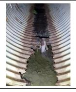
Aging Infrastructure – underground road drainage pipes are at the end of their useful life and are starting to fail at an increasing rate. Some of the failures lead to sink holes in the roadway.
