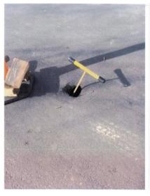
Sinkhole in the roadway caused by road drainage pipe failing. We currently have a sinkhole on Hazel Avenue in East Richmond Heights. Several years ago we had a sink hole form on Marsh Creek Road that required immediate action to prevent the lane from collapsing.
