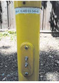
Cathodic protection test point along the Iron Horse Corridor
