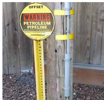
Multiple utilities exist in the Iron Horse Corridor
