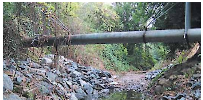
Examples of other pipelines crossing steam areas in California and Washington States.
