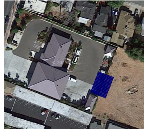
Fire Station 84 Pittsburg 33 kW
