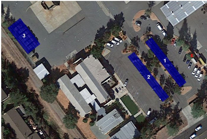
Fire Station 10 & Training Campus Concord 135 kW
