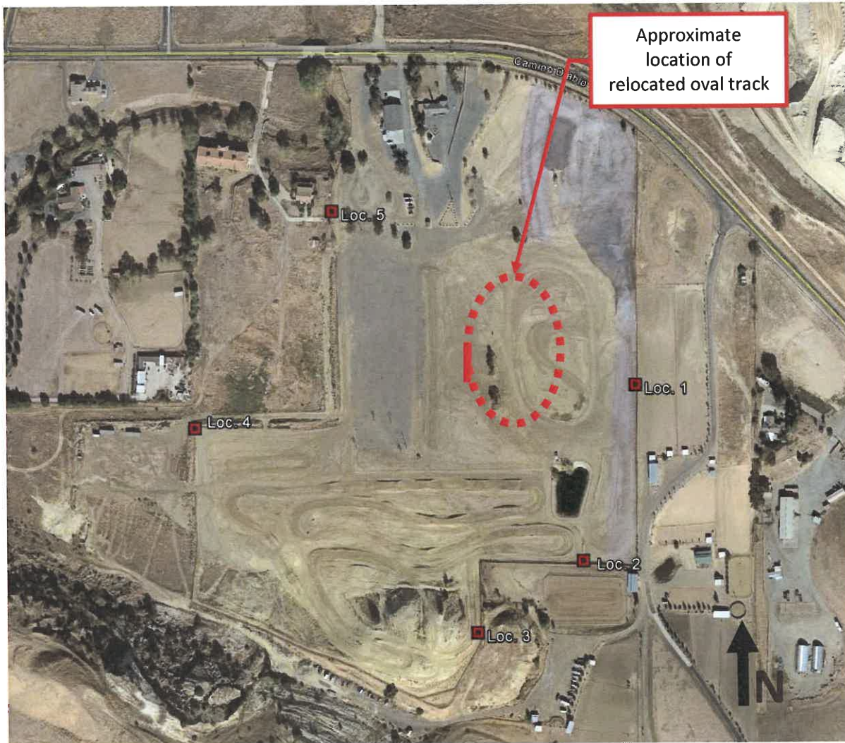
Figure 1: Aerial View of DMXR Facility Showing Noise Measurement Locations
