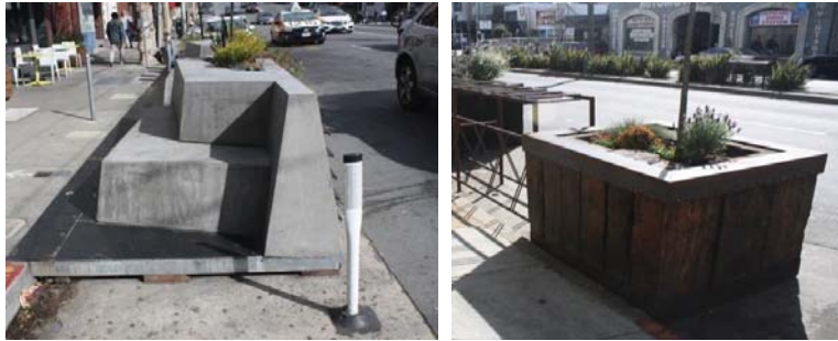
Figure 9: Samples of Fortified Railing/Barrier
