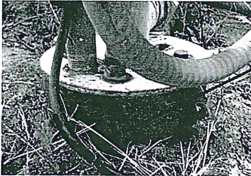
Figure 3 – Entry Point for Contaminated Water to Reach the Aquifer (DWR)
