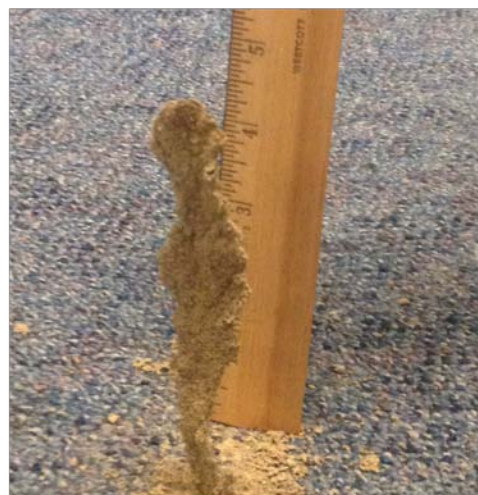
Subterranean termite tube emerging from a crack in the slab under the carpeting of a ground floor hallway at 597 Center in Martinez
