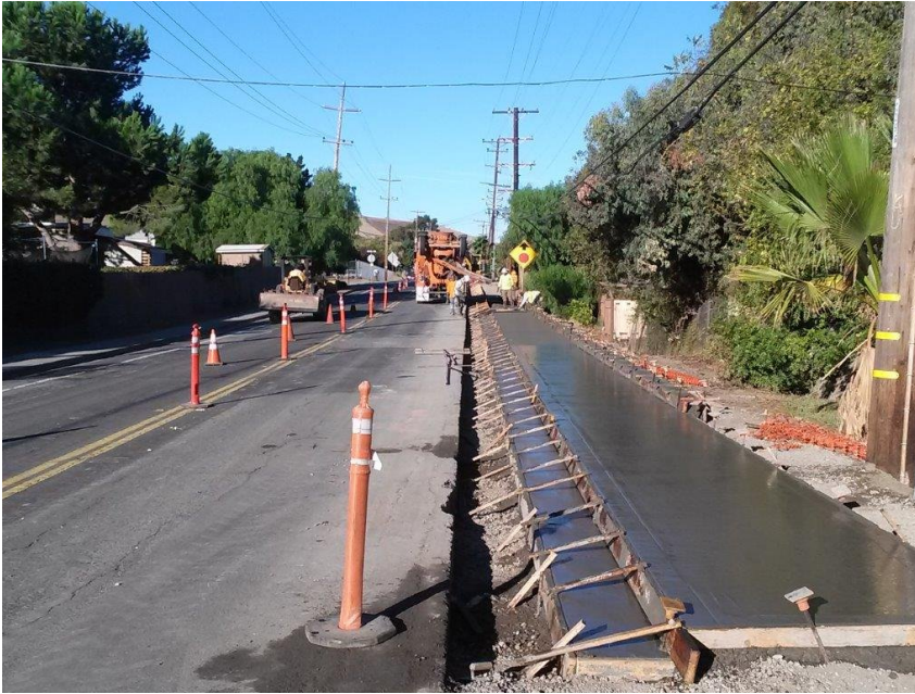
New Sidewalk Being Constructed
