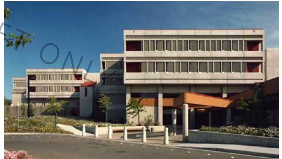
Figure 2: Exterior view taken shortly after construction completion.
