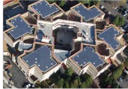
Figure 4: Aerial view of the MDF facility.
