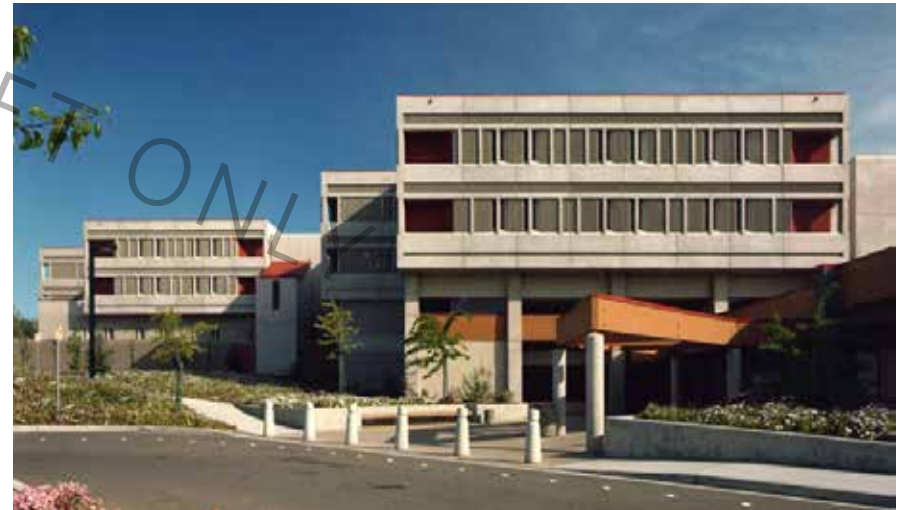
Figure 2: Exterior view taken shortly after construction completion.
