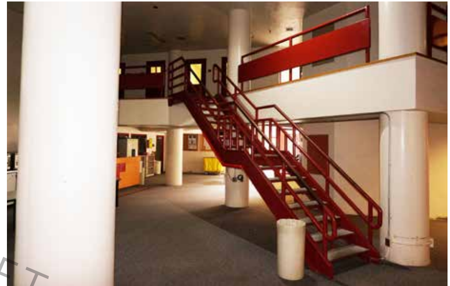
Figure 37: The typical housing unit is irregularly planned and has large structural concrete columns throughout making supervision from one point impossible.
