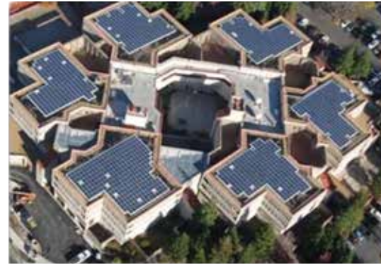
Figure 4: Aerial view of the MDF facility.
