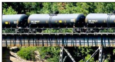
A crude oil train travels across the Clear Creek Trestle in Plumas County, California and through the Feather River Canyon on June 5, 2014.
