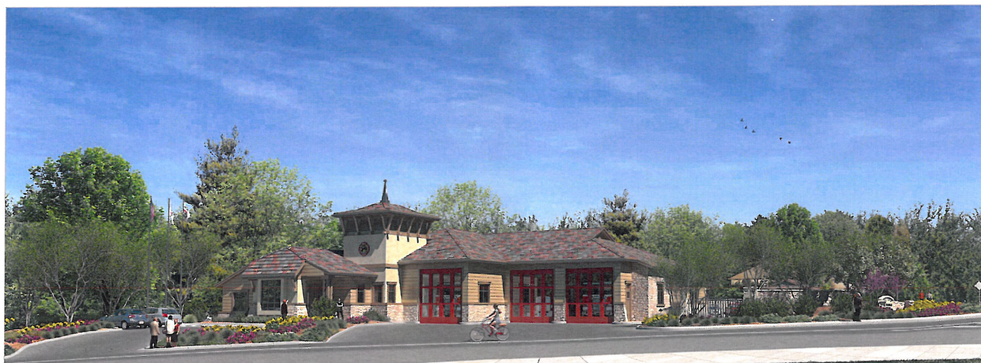
② VIEW ALONG MIRANDA AVENUE
