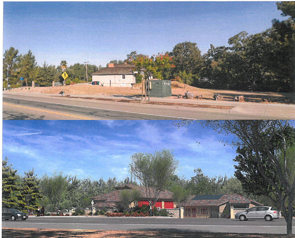
1 VIEW ALONG STONE VALLEY ROAD
